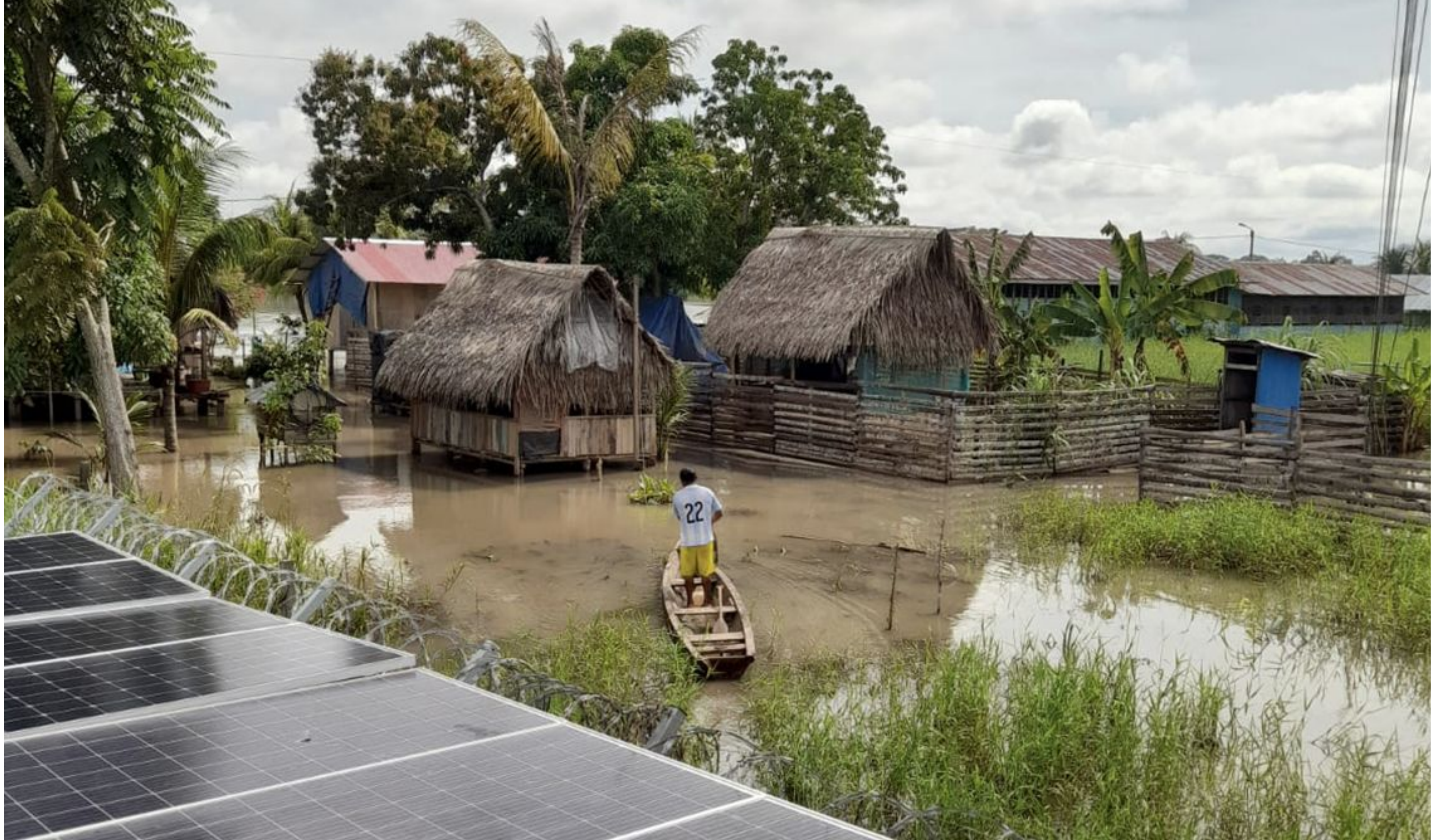
Getting off Diesel with Project SIEMIC in offgrid locations ( link )
